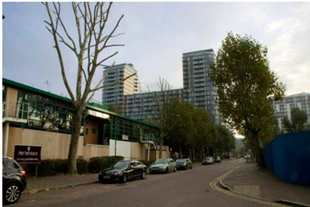
Existing View from North-West of Building
